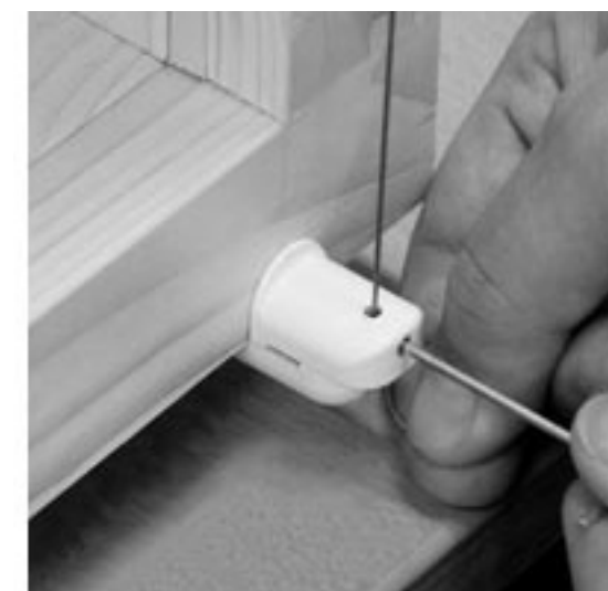
c. locking guide wire
